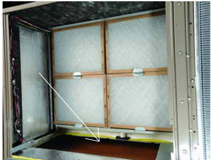
Figure 16: Bottom supply opening for side duct conversion
