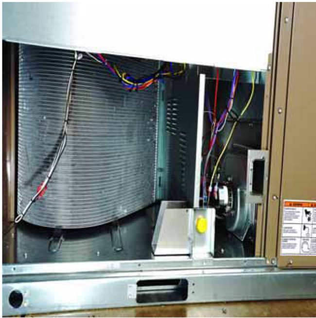
Figure 22: Flue exhaust hood installed
