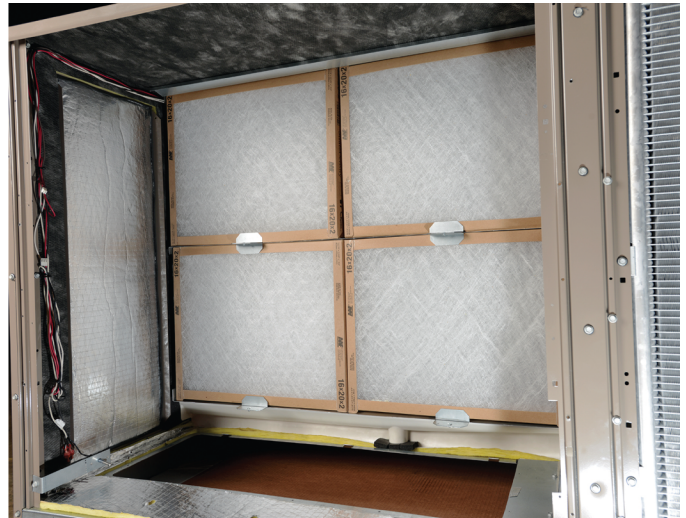
Figure 15: Bottom supply opening for side duct conversion
