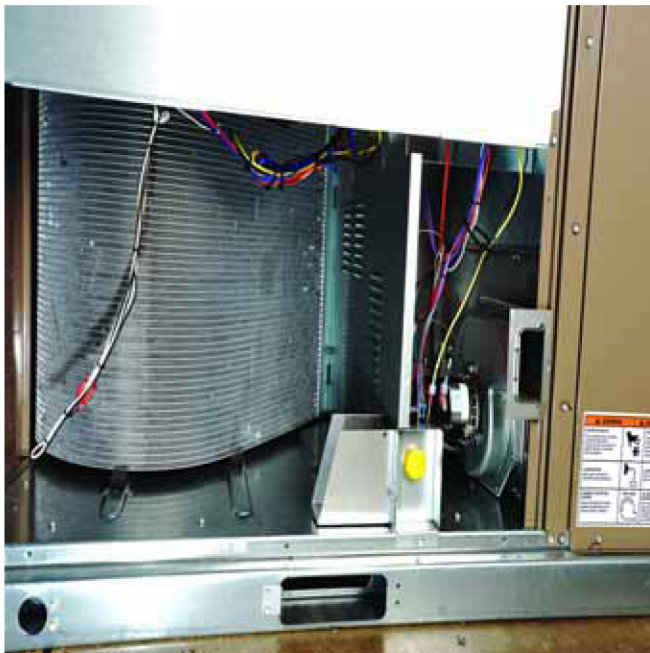
Figure 22: Flue exhaust hood installed
