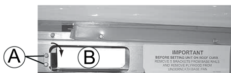
Figure 1: Unit shipping bracket
