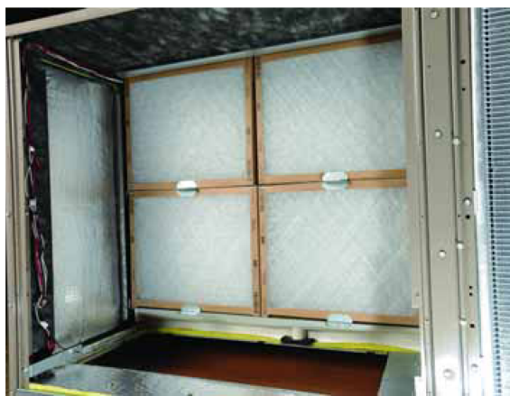
Figure 15: Bottom return opening for side duct conversion
